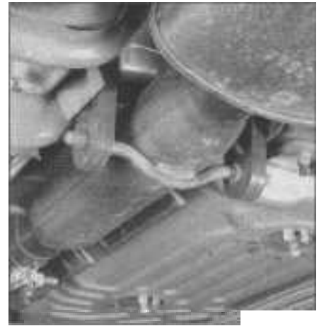
18.1 Inspect the exhaust system mounting brackets, clamps and rubber hangers for damage or improper installation
