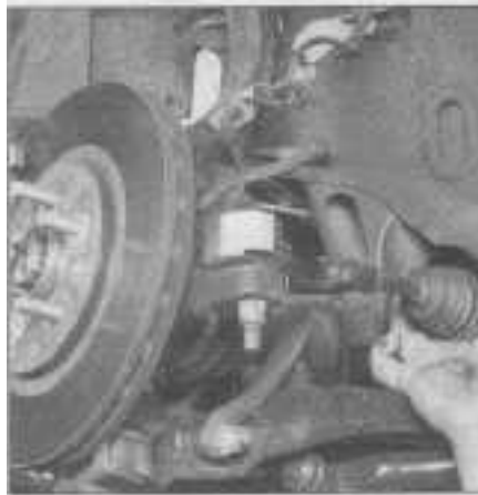
14.5 Checking the steering rack tie-rod boot for damage
