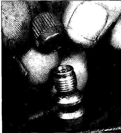
The protective cap on service valves performs two functions - it keeps the core clean so no contaminants get into the system when the service valve is open and it prevents accidental discharge of the system if the core fails
